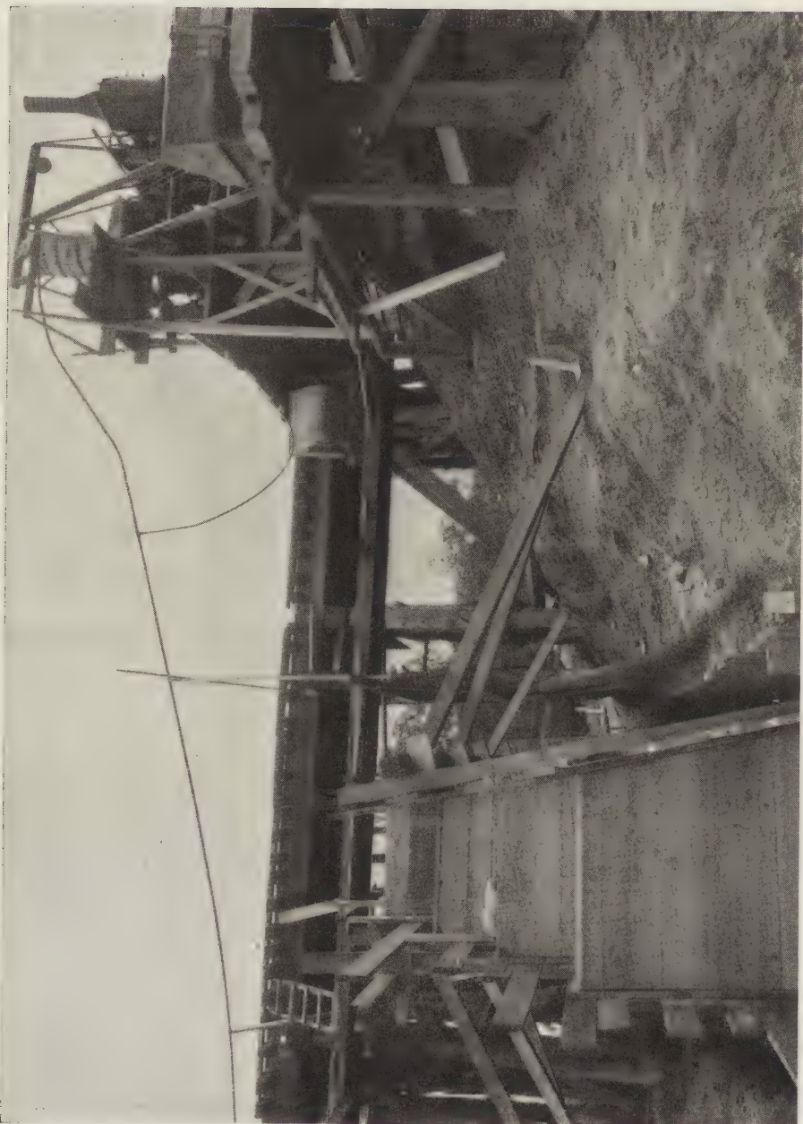
Fig. 20.—View showing method of transporting and placing concrete for railroad bridge abutments.
